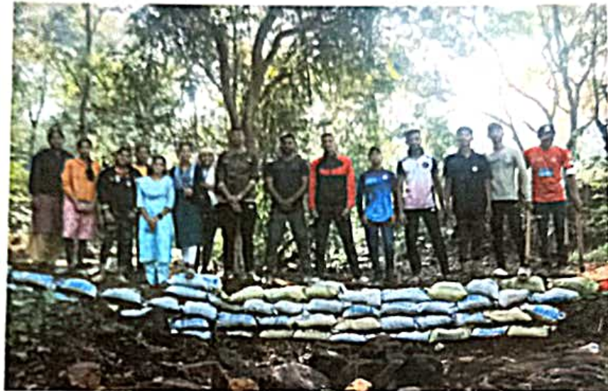
Construction of Bunds in Adopted Village
